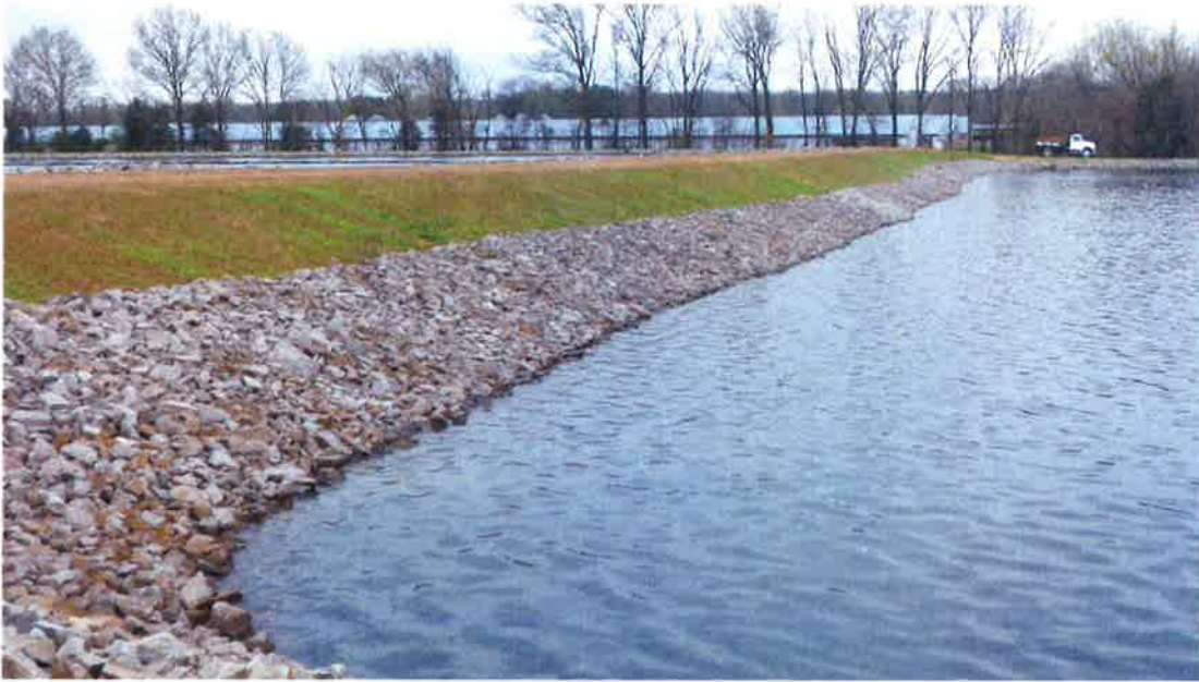
Photo 1 Rip Rap and Stabilized Levee West Shore of Lagoon 3
