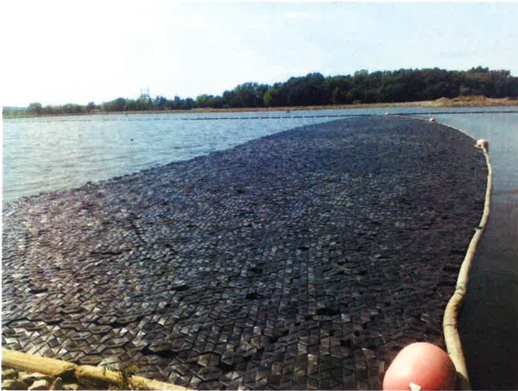
Photo 2 Hexprotect Floating Cover Tiles Contained Using a Temporary Floating Baffle
