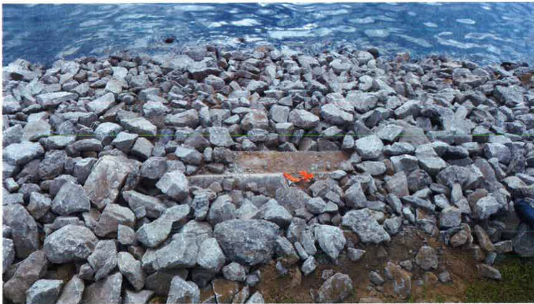
Photo 4 Mooring Block and Loop for Baffle Curtain West Shore of Lagoon 3
