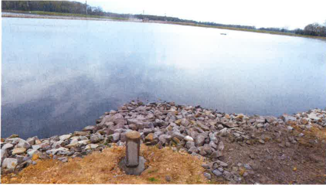
Photo 5 Bollard and Rip Rap for Baffle Curtain East Shore of Lagoon 3
